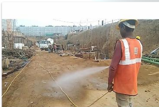
Figure 4b: Dust mitigation measures are taken at the under-construction area of Aerocity
