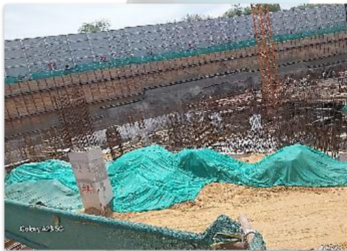
Figure 3 a: Dust mitigation measures are taken at the under-construction area of Aerocity
