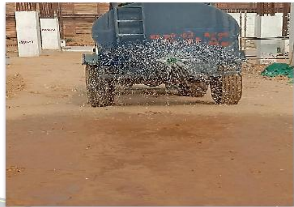
Figure 4c: Dust mitigation measures are taken at the under-construction area of Aerocity
