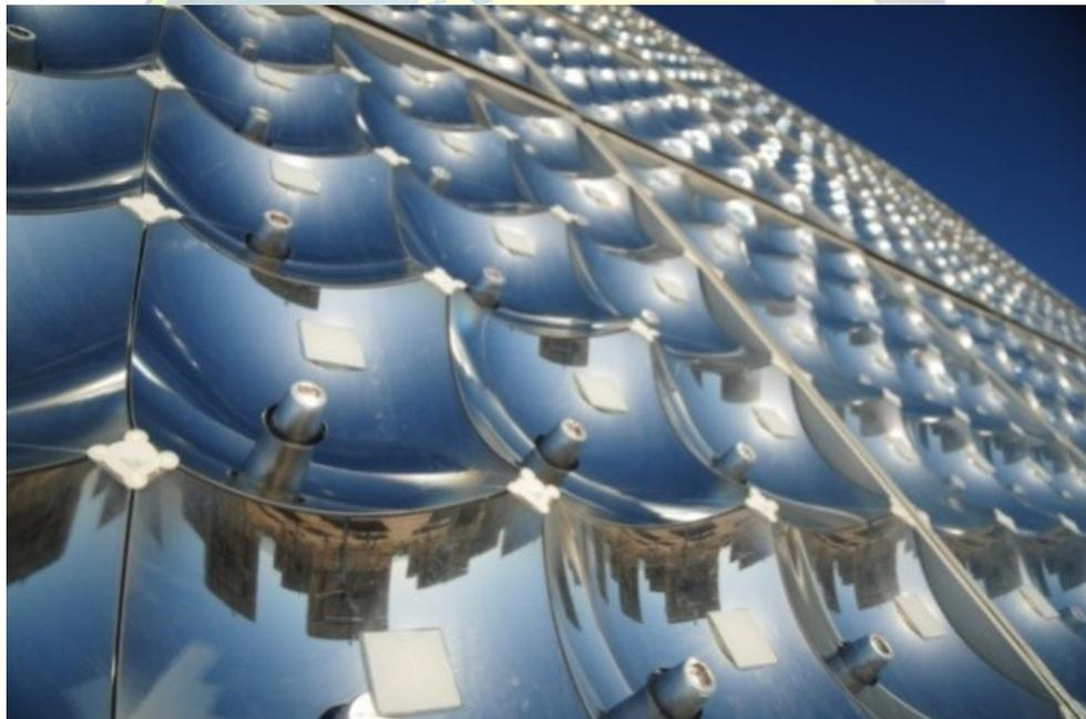
Due to the recent drop in Si solar module prices the concentrator solar modules are not commercially viable.
