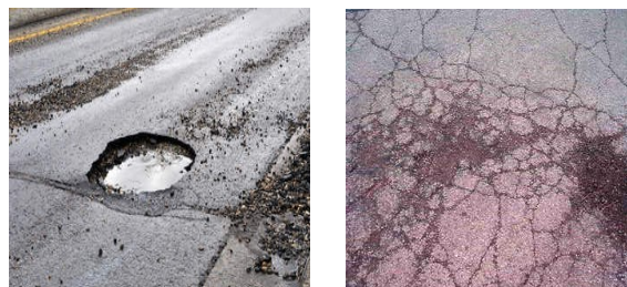
Figure 1: Asphalt pavement defects (a) Potholes (b) Cracks
