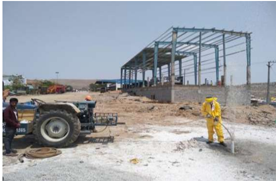
Fig. 3. Flashing of recharge well during initial installation
