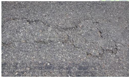
Fig.2. Figure shows the various surface defects on the road surface captured through 'share app'
