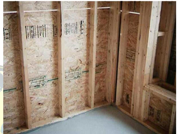
Fig Plywood shear wall
