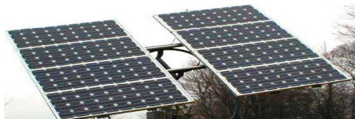
Fig. 2. Dual Axis Tracker
