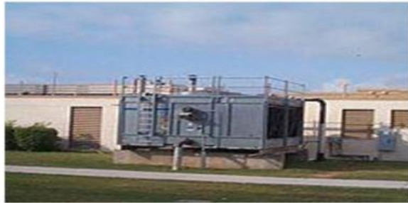
Fig: Mechanical draft cross flow cooling tower used in an HVAC application
