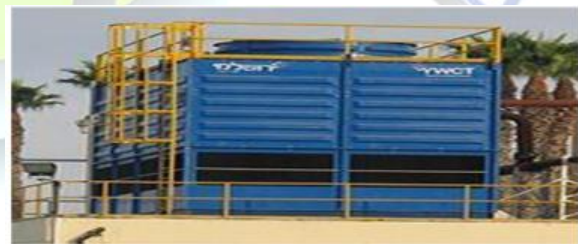
Fig: Forced draft counter flow package type cooling towers
