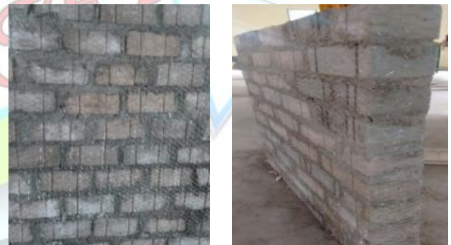
Figure-2.4 Confining of brick walls
