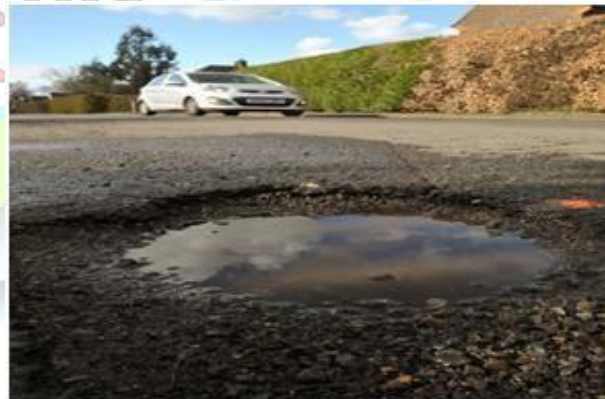
Fig. 1. Condition of roads with potholes.
