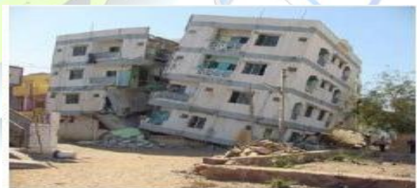
Soft Storey (Open Plinth), Vertical Split between two blocks (Bhuj)
