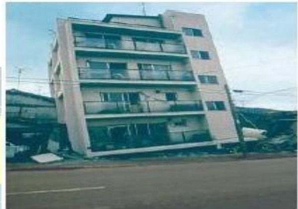
Soft first storey collapsed, upper part of the building fall onto the ground, (Kachchh, 2001)
