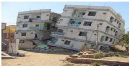
Soft Storey (Open Plinth), Vertical Split between two blocks (Bhuj)
