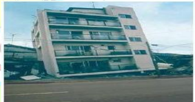
Soft first storey collapsed, upper part of the building fall onto the ground, (kachchh, 2001)
